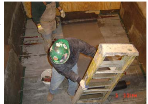
Installation of Rawmat HDB prior to placing concrete
