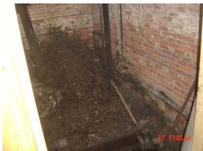
Elevator pit prior to waterproofing
