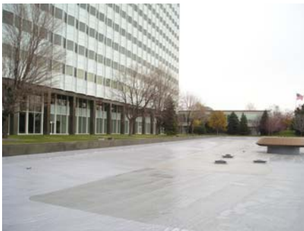
The polyurea liner was terminated along concrete edge wall
