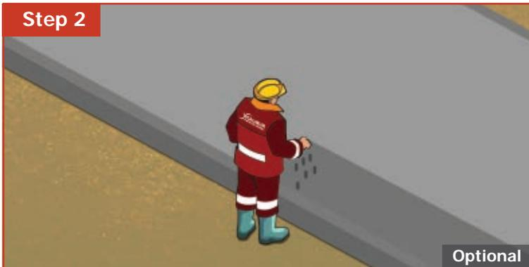
After bleed water has evaporated, immediately reinforce edges by spreading hardener by hand along a 150 to 200mm edge and finish using wooden trowel.
