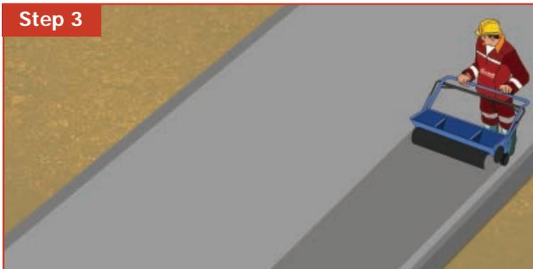
Immediately the concrete can take a mason's weight (slight foot imprint <3mm). Use a dry shake spreader and spread approx 50% of X-Tech IntegraFloor.
