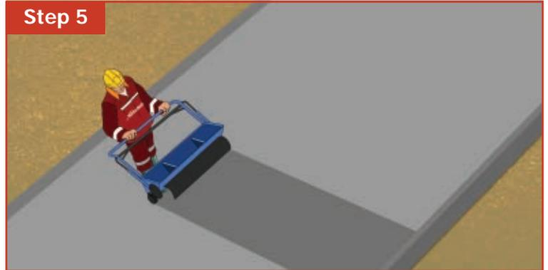
As soon as Step 4 has started follow with the second application of X-Tech IntegraFloor. Apply at a right angle to the first application.
